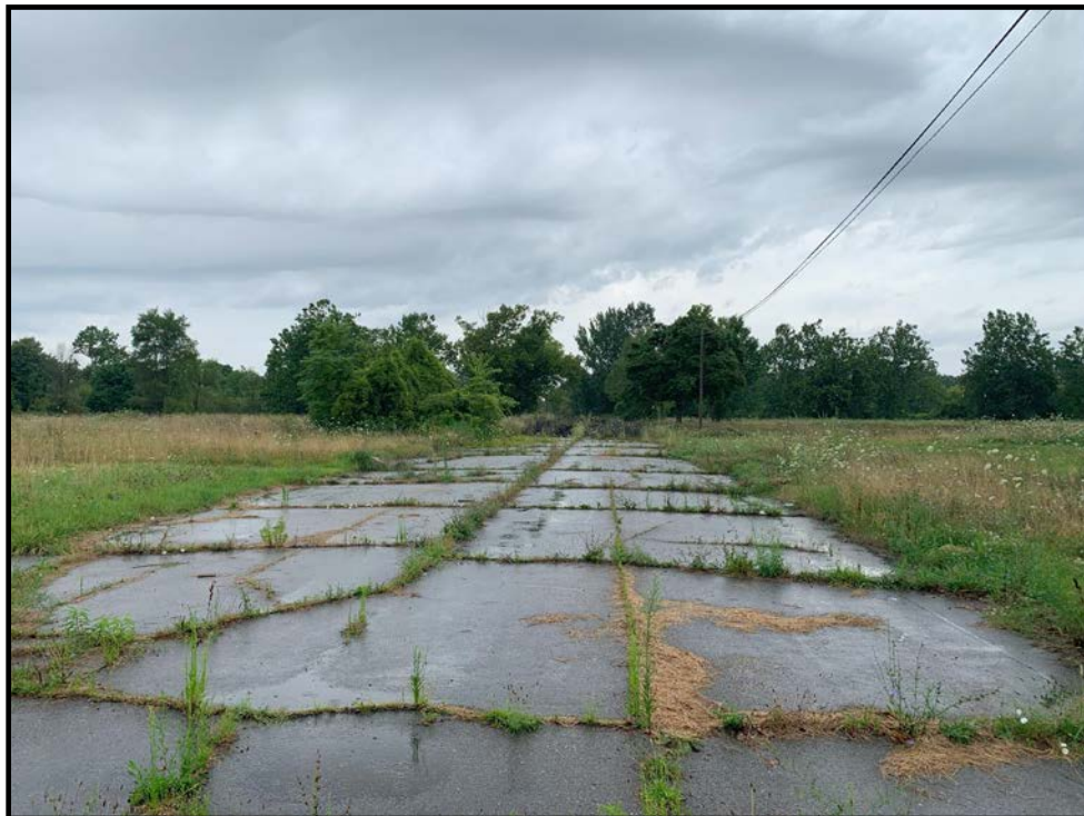
Photo 6: View of Frankfort Court road easement which bisects the subject property.
